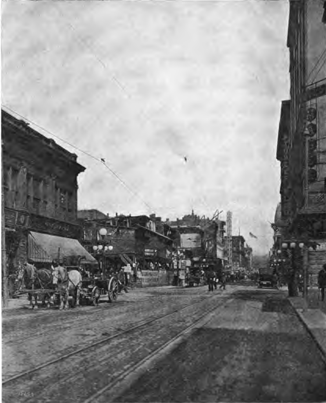
Robert Street, St. Paul, Minn. Front of buildings torn down for widening of street
